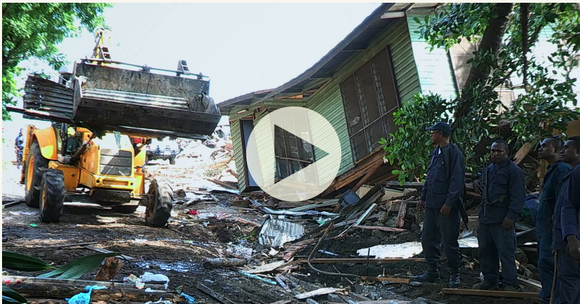
THE OPPOSITION CLIP 01: DEMOLITION
